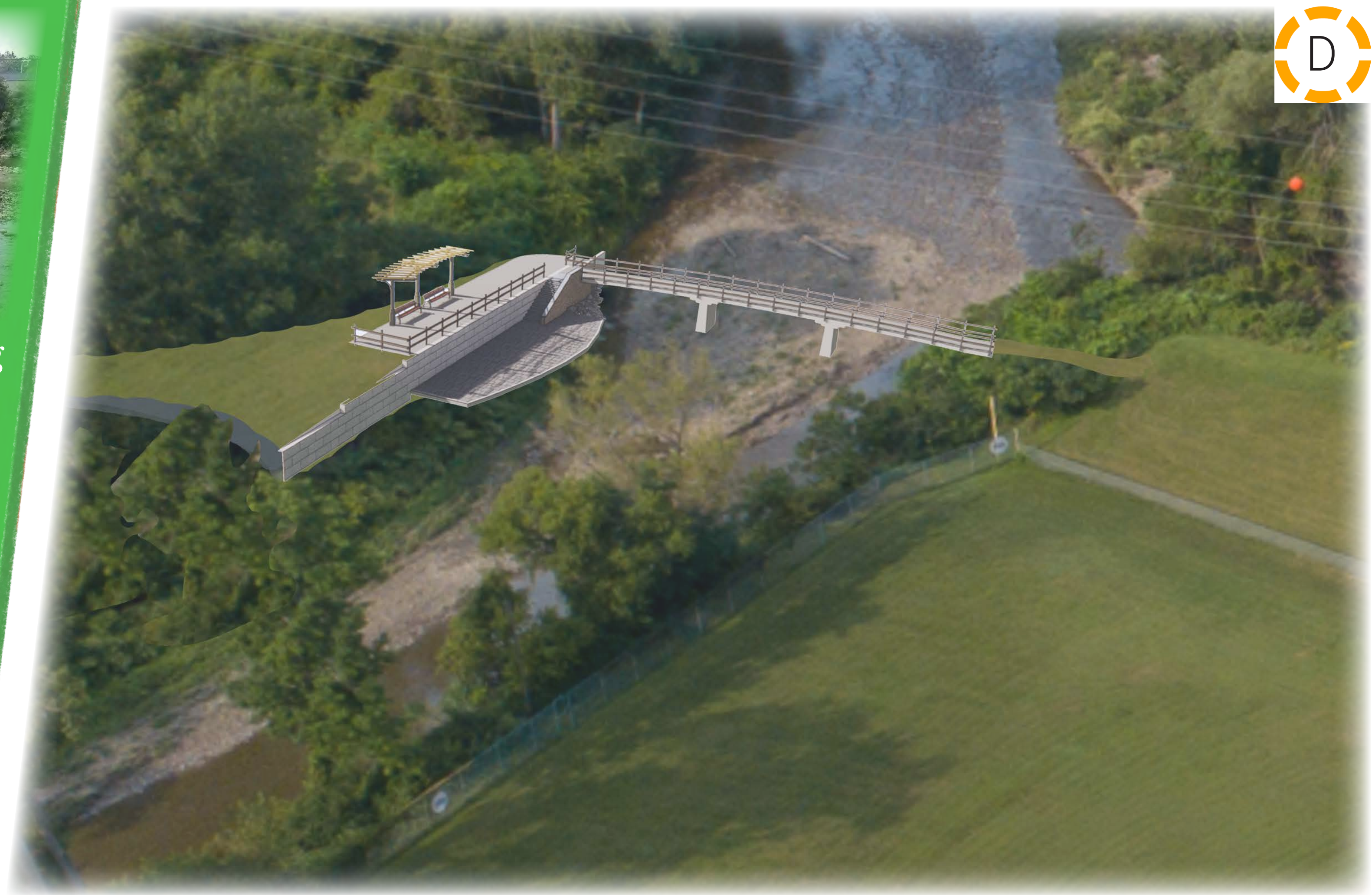
Aerial View Displaying Cold Creek Footbridge
