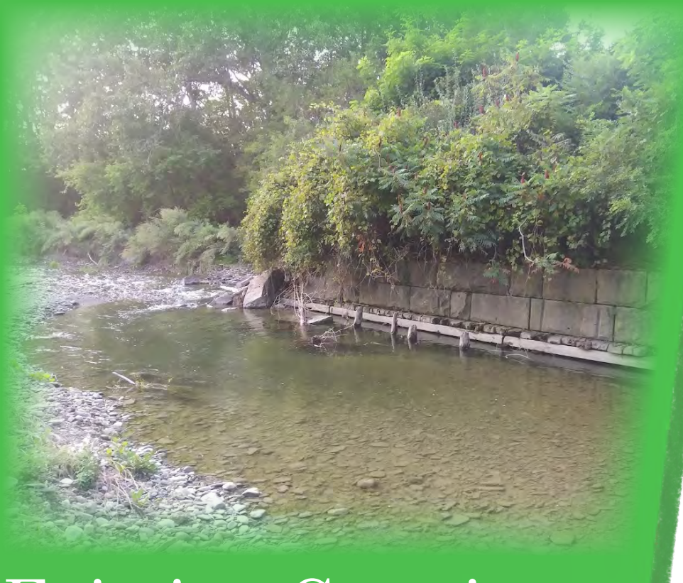
Existing Crossing North Bank
