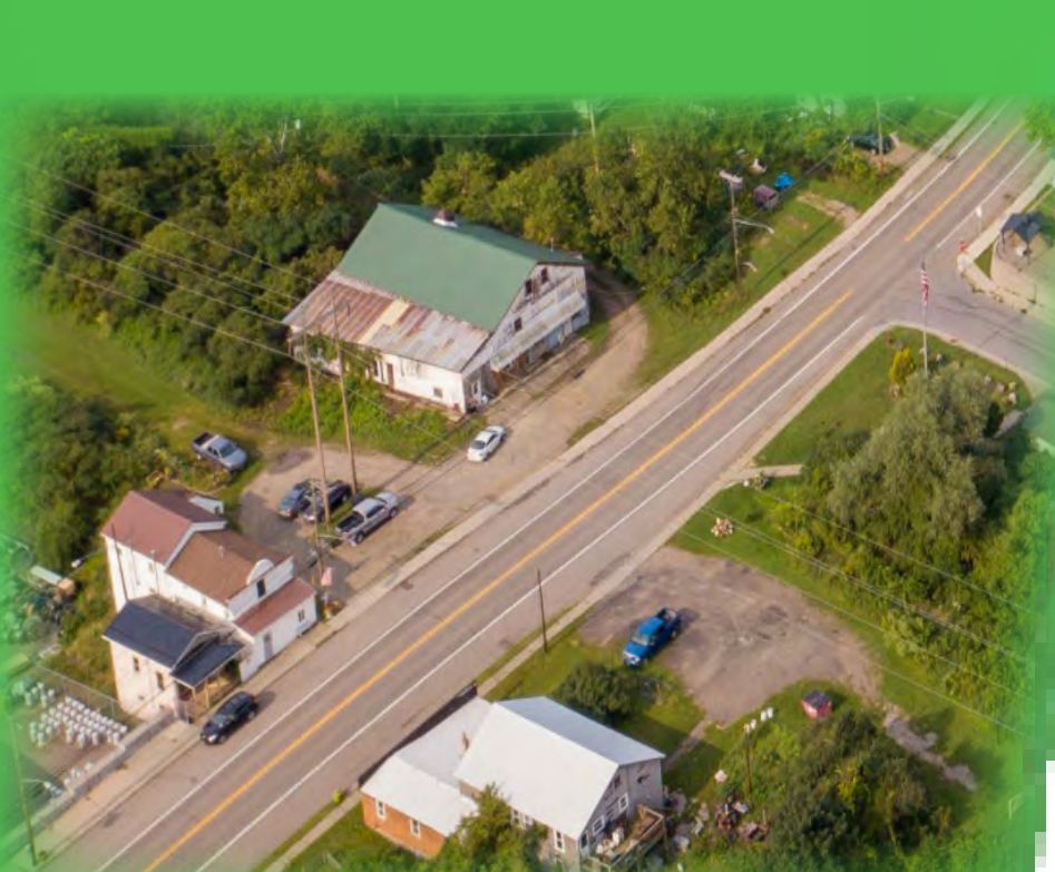
Existing condition of Genesee Valley Greenway site.
