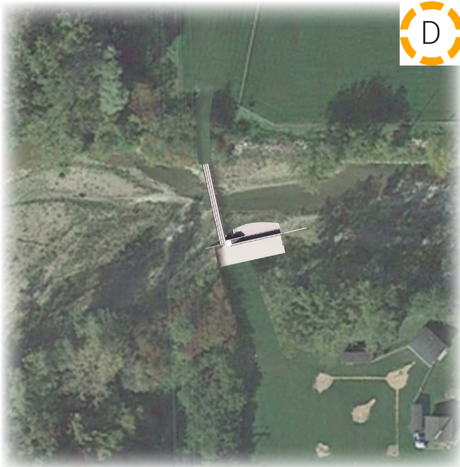
Cold Creek Foot Bridge
