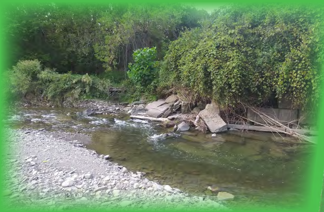
Existing Crossing North Bank
