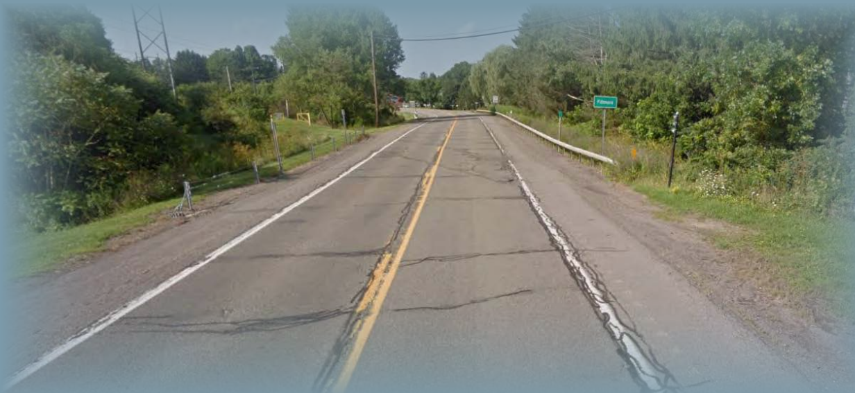
Genesee Valley Greenway Intersection on Route 19
