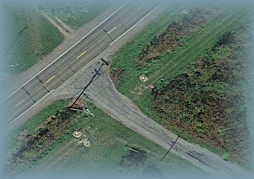
Birds Eye View of the Greenway & Lattice Bridge Road Intersection
