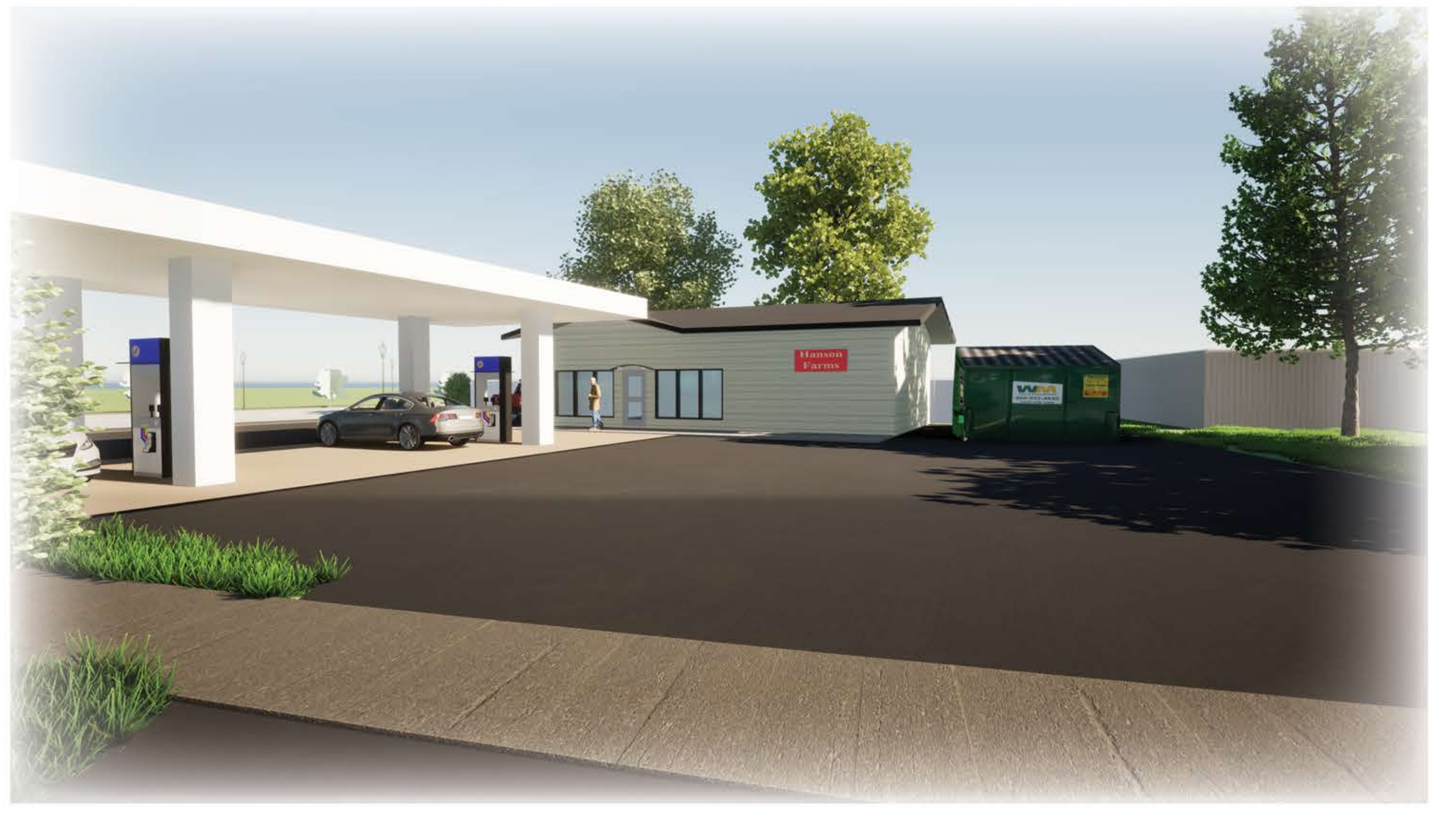
Front View from South Genesee Street
